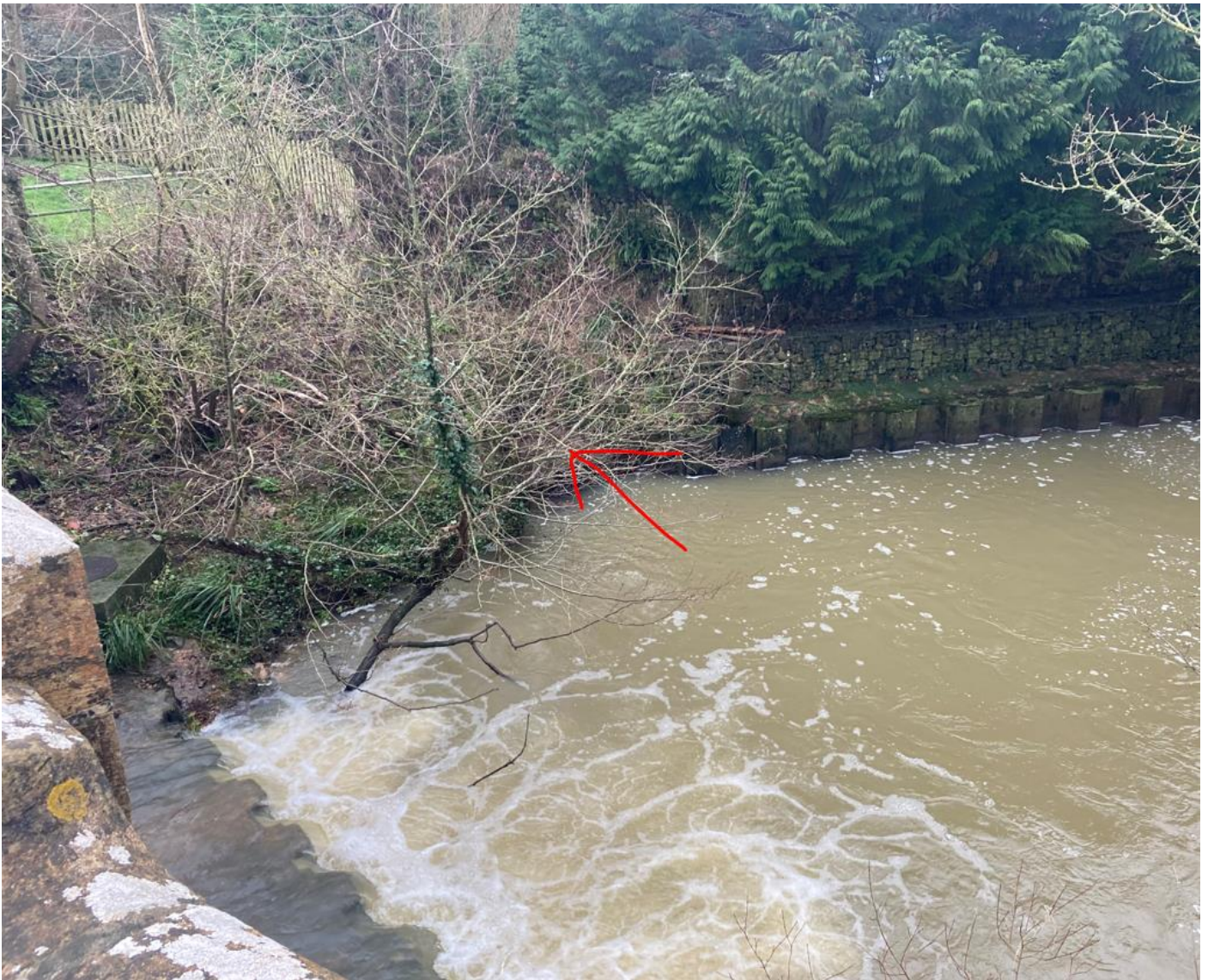
The outfall to the river (no overflow contributing today)
